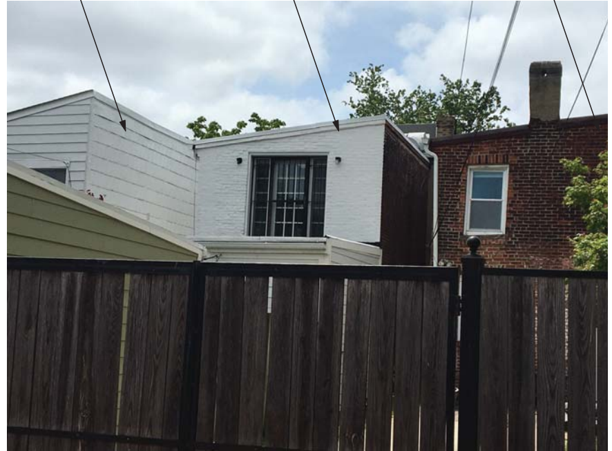
Rear elevations from Alley
