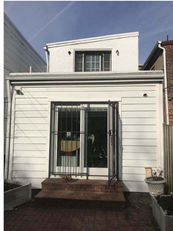
Rear Elevation of 514 9th St. with existing 1-story Kitchen addition
